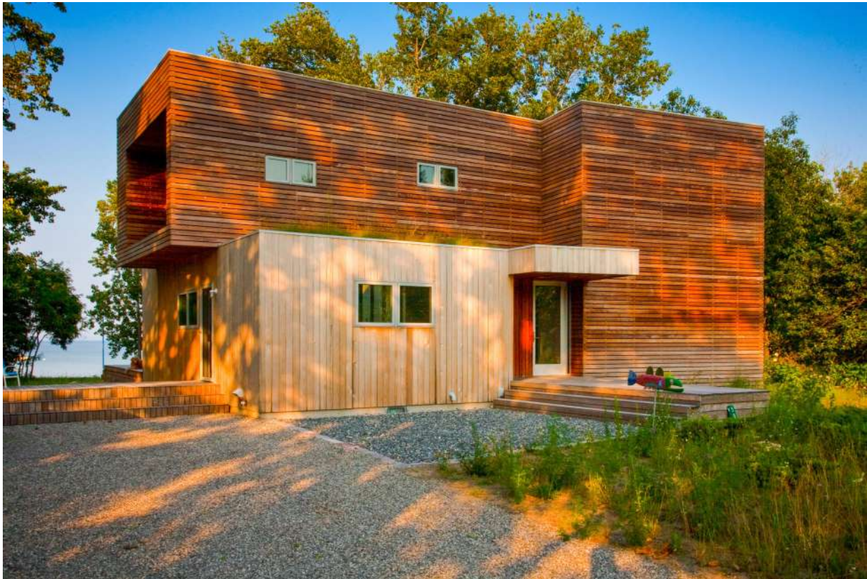
Figure 5: The natural shading is clear in this image. Another part of the solar deflection strategy was the Ipe-clad rain screen.
